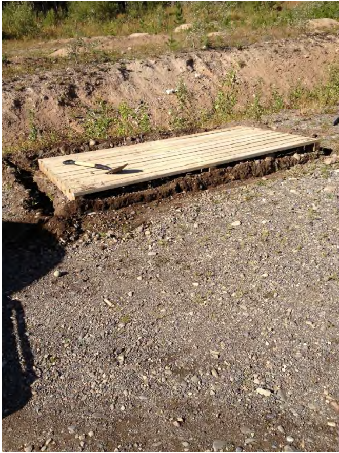
Figure 1: Frame and Catchment Pit
