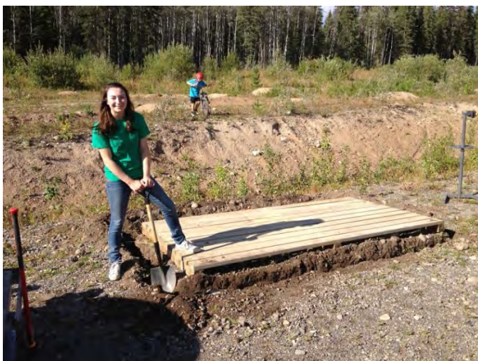
Shelby Longstaff Digging the Cathment Pit.
